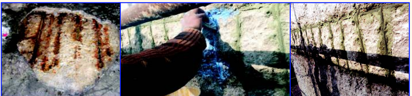
Corroded Section get treated at Fertilizer Plant, Visakhapatnam
