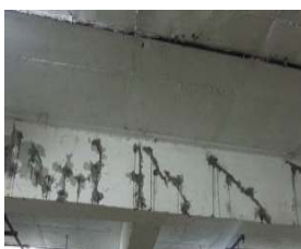
Injection Grouting
