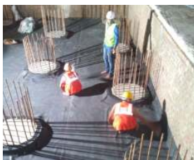
Membrane Waterproofing
