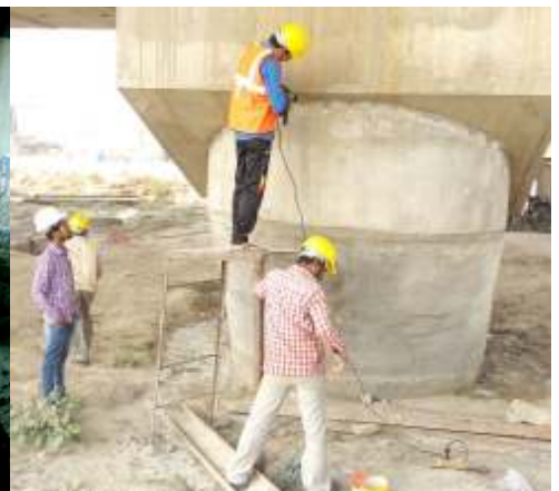
Injection Grouting over Bridge at Bihar
